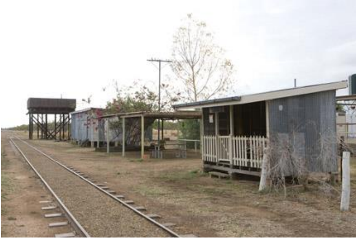
Blackbull Siding, Normanton-Croydon Railway Line
