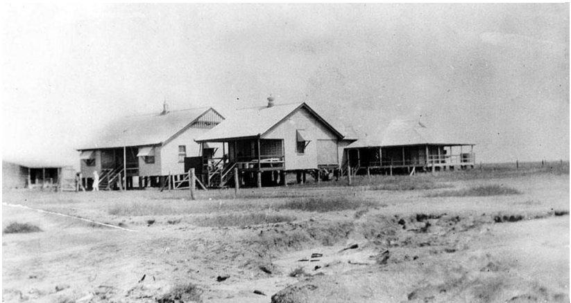
Burketown Hospital, 1924 (State Library of Qld, negative number 46495)
