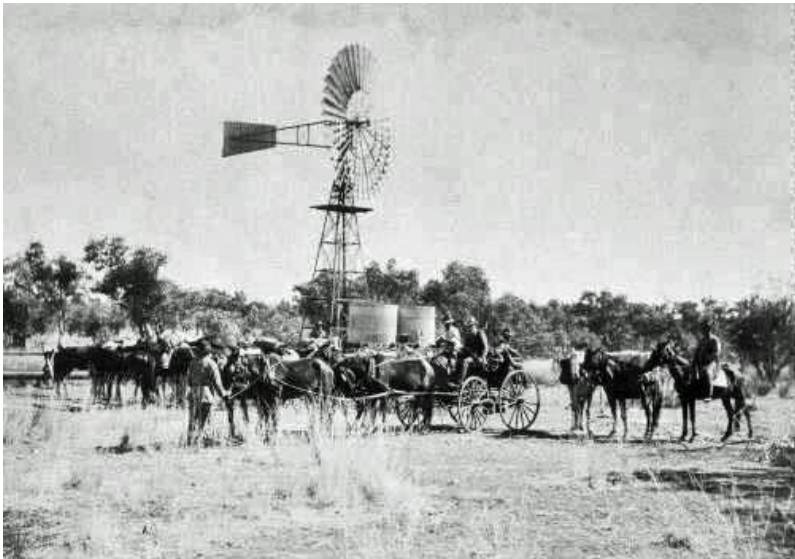
Work on Overland Telegraph Line, 1919 (Territory Stories, NT Government, photo PH0820/0070)
